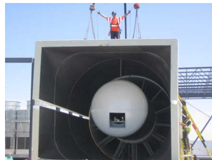
Figure 8.10: Air circuit elements and main fan being assembled on site.
