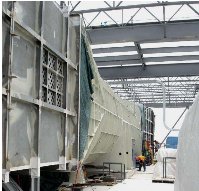
Figure 8.11: 3 rd floor building level, viewed from corner 2, showing fan anchored to portal frame, with transition sections to each corner.
