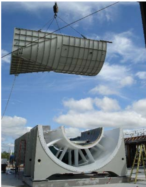
Figure 8.10: Air circuit elements and main fan being assembled on site.
